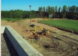
West track area
