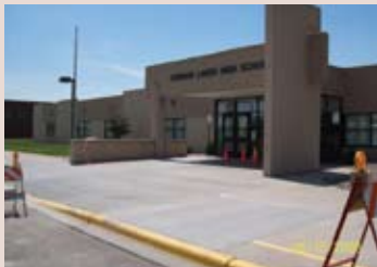
New front entry sidewalk is complete at the High School.
